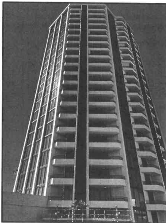
Photograph #2: Completed scope of work at the 04/05 balcony stack
