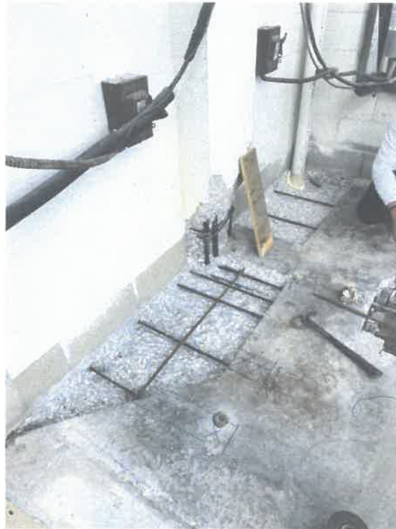
Photograph #1: In-progress column and slab repair at Unit 1A4/library AC closet
