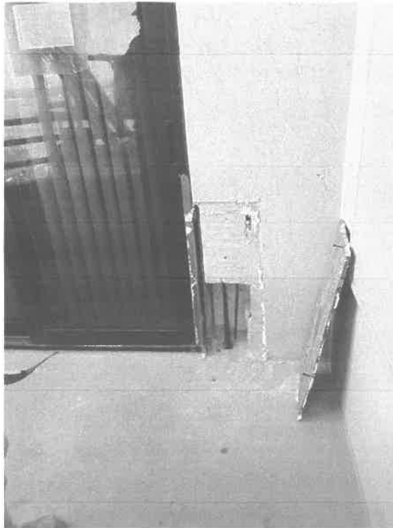
Photograph #1: Completed wall repair at the 01 balcony stack
