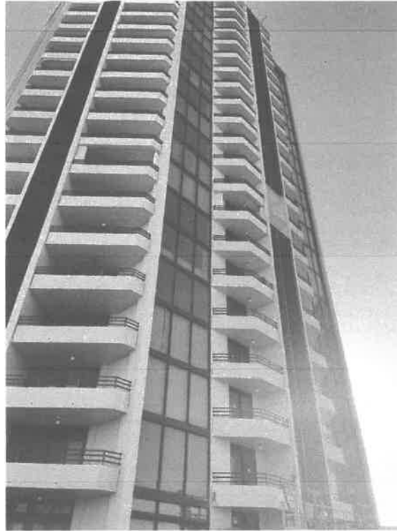
Photograph #3: Inspected repairs at the 01/06 balcony stack of Tower A
