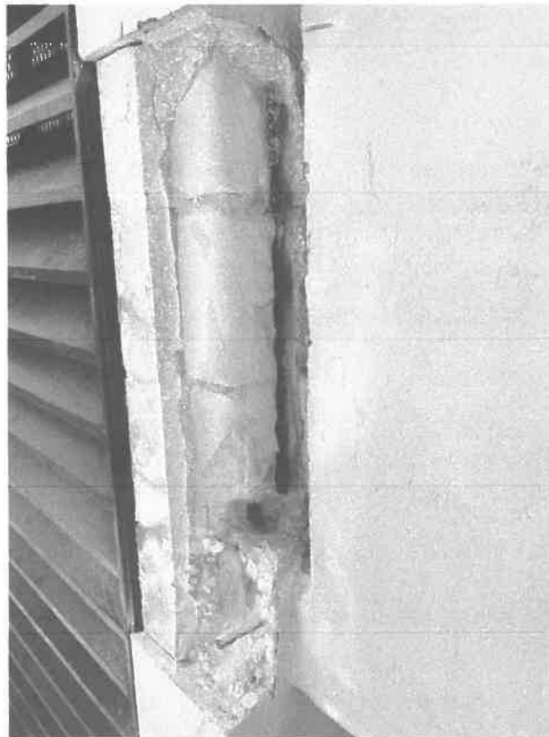
Photograph #4: In-progress repair excavation 01/06 stack wall
