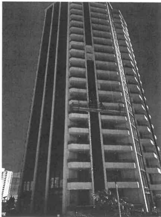
Photograph #2: Concrete repair in-progress at the 01/02 balcony stack
