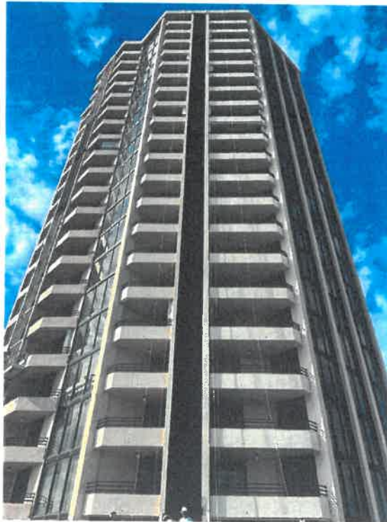
Photograph #2: Completed scope of work at the 02/03 balcony stack
