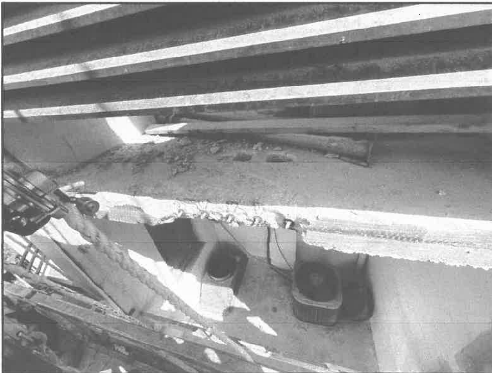
Photograph #2: In-progress post tension repairs at the 01/06 balcony stack.
